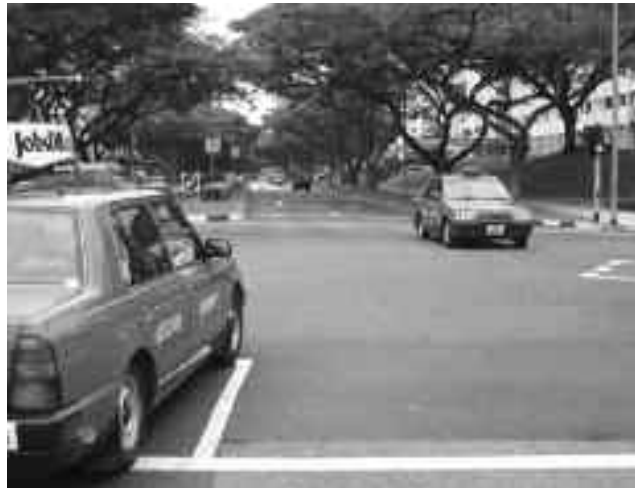
Figure 3: Before treatment: vehicles waiting at the right-turning pockets for a gap to make a right turn
