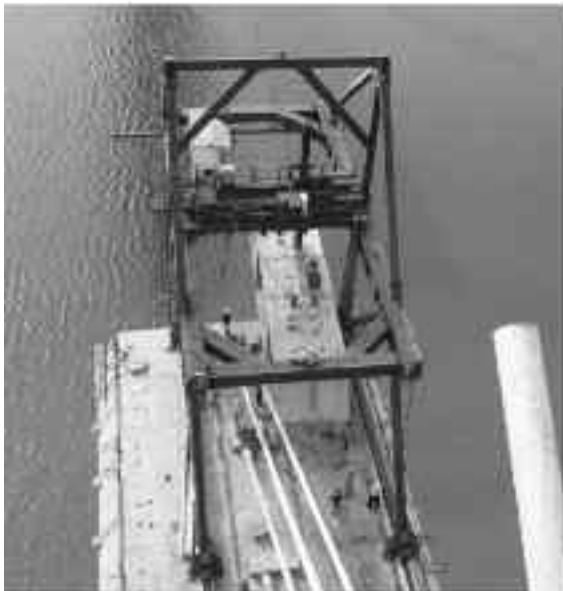
Figure 6: Lifting of cable stay segment using 'A Frame'
