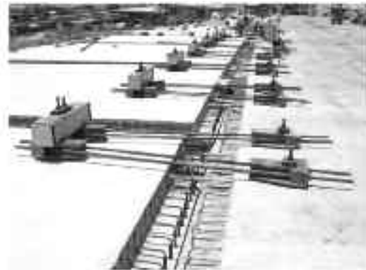
Figure 11: Temporary clamping devices for side frame
