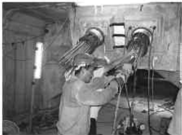
Figure 7: Stressing of stay cable strands using monostrand jack
