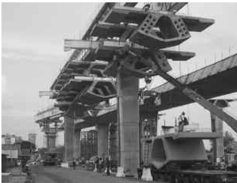
Figure 8: View of 400 tonne small launching gantry for erection of ramps
