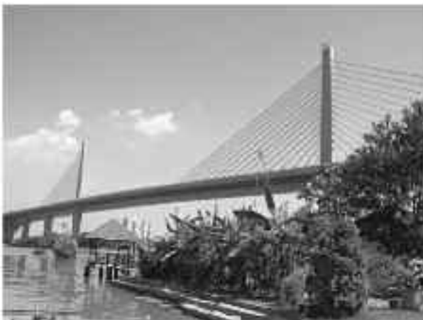
General view of Sungai Prai Bridge
