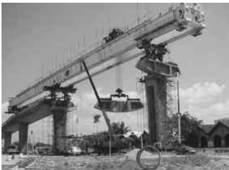
Figure 5: Overview of 880 tonne overhead launching gantry (1500 tonne capacity)
