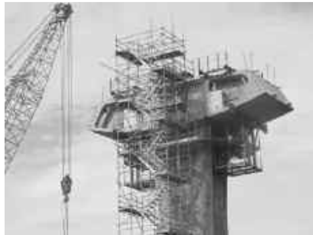
Figure 4: Steel bracket supported the pier head segments
