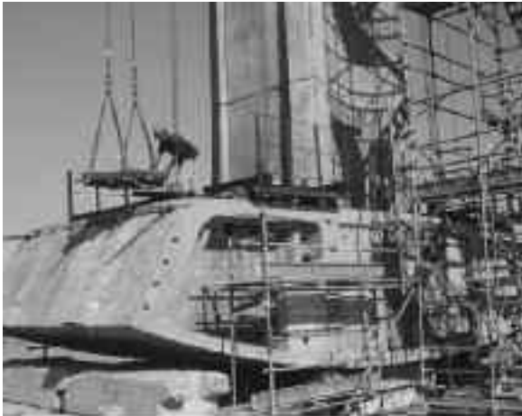
Figure 3: Adjusting pier head segments before lifting
