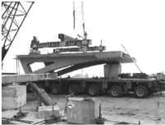
Figure 10: Lifting of side frame using mobile crane
